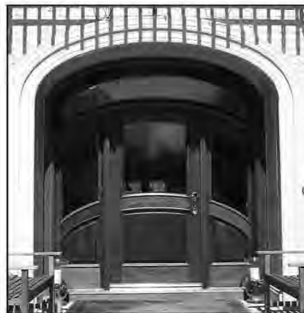
Custom door designed and built by TW Perry
