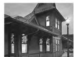
Tuxedo Station Tuxedo, NY
